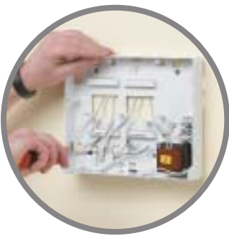
Mounting pulling cable through and wiring the Panel
