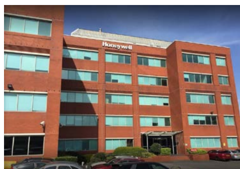
The Bracknell training Facility
