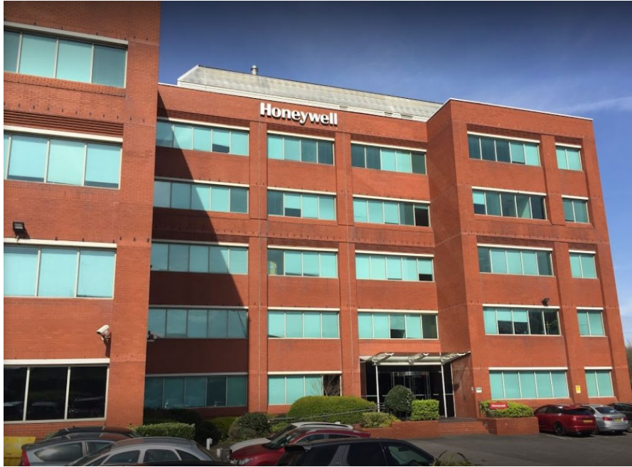
The Honeywell Bracknell Office
